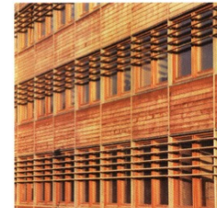
WRC cladding (now turned silver grey) for the New Jubilee Campus, Nottingham University (opened 1999) by Michael Hopkins and Partners; MHP 1999.
