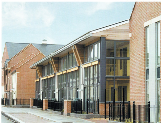
The ZED Housing development built to meet Code Level 6 using the ruralZED™ zero carbon housing system in Northampton.
